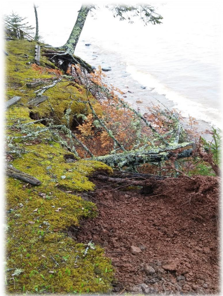
South Shore Erosion Damage
